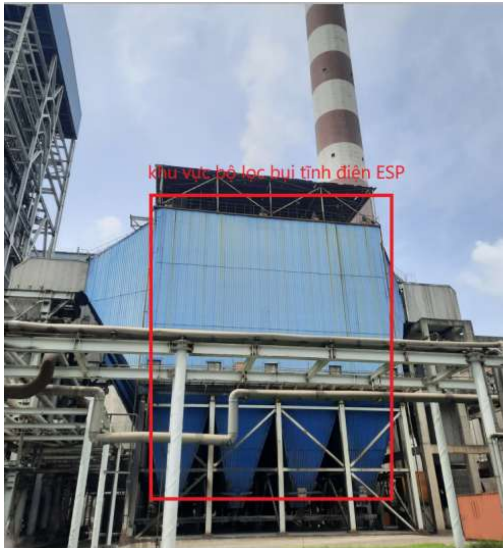
Figure 3.5: Image of the ESP electrostatic precipitator area
