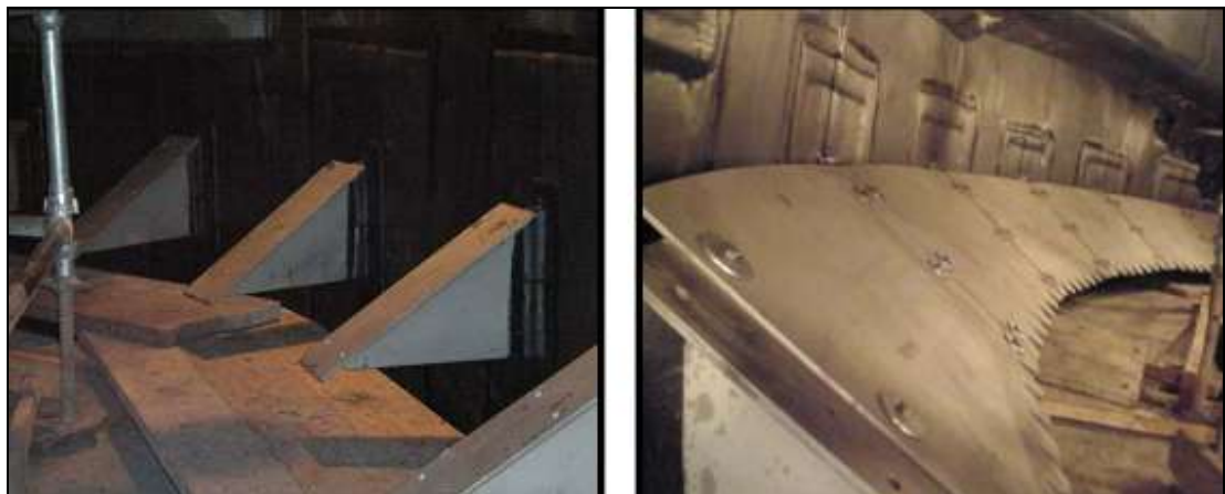
Figure 2.3.6: Installation of baffle rings at Unit 2, BL England power plant.
