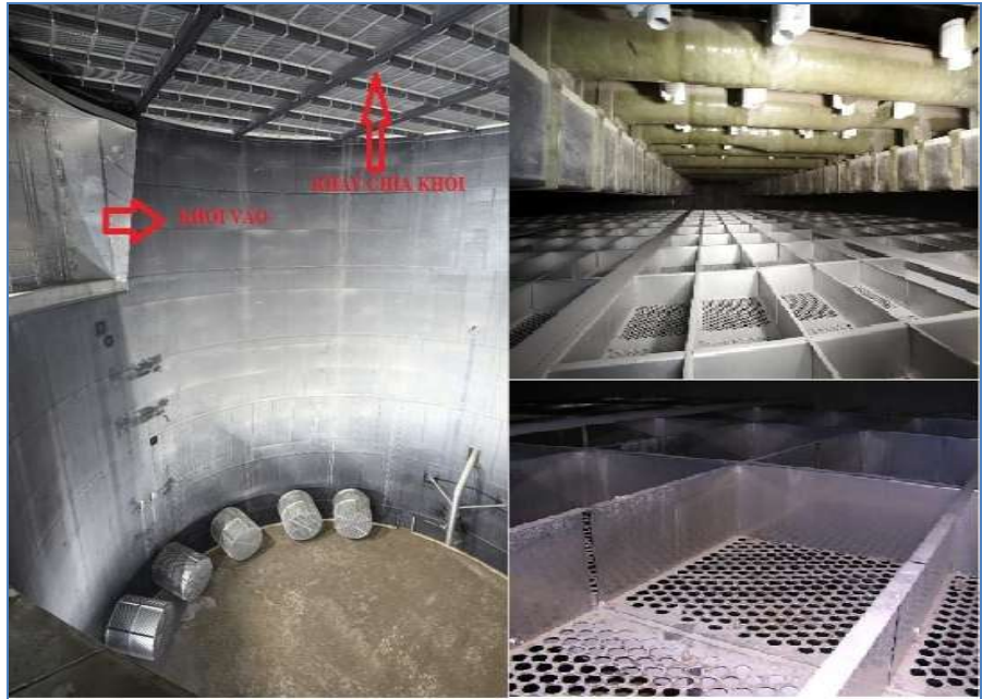
Figure 2.3.9: Position and shape of the newly installed induced draft splitter tray.
