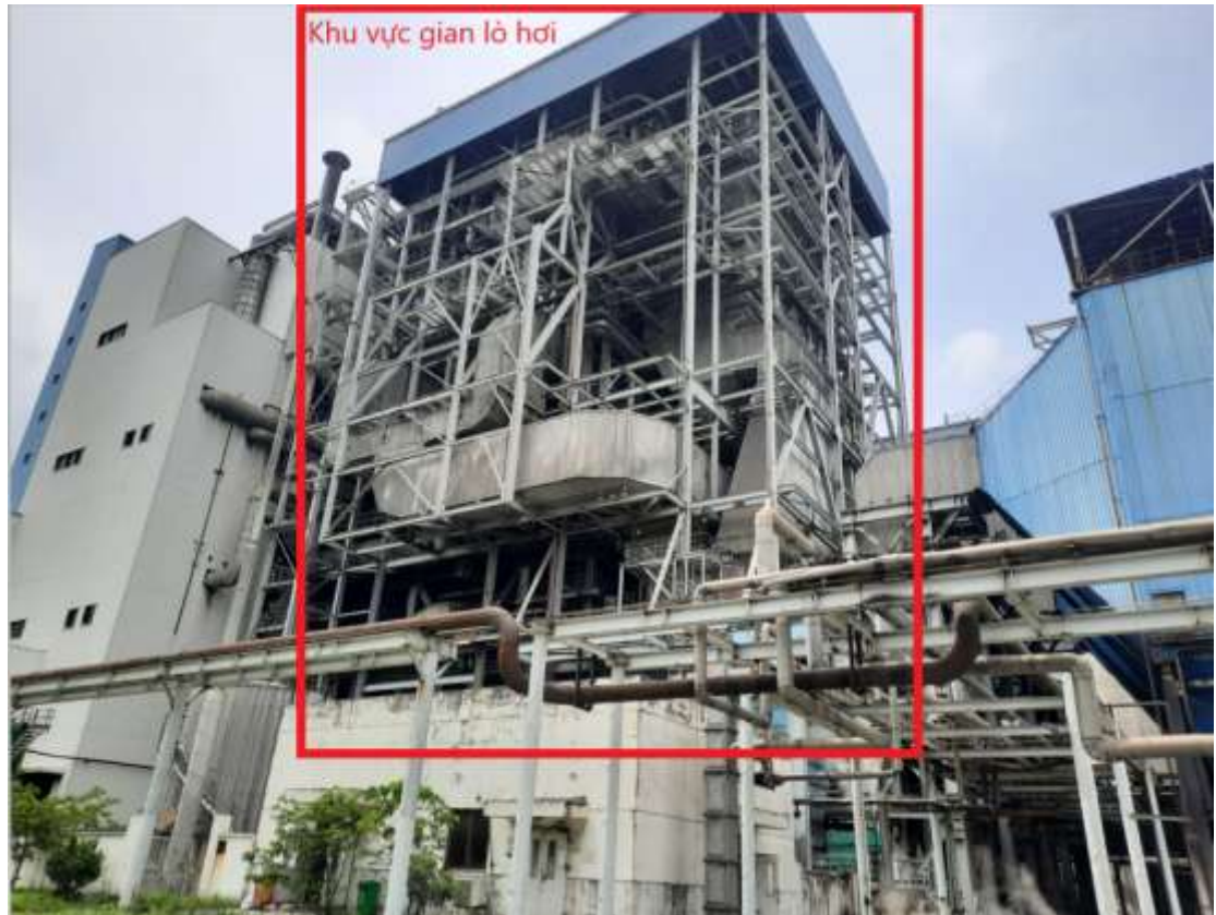
Figure 3.1: Current status image of the boiler room area
