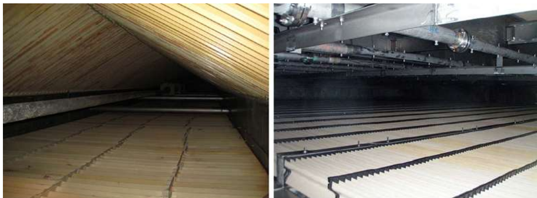
Figure 2.3.13: Upgrading the nozzle and flue gas distribution tray at the Fayette power plant.
