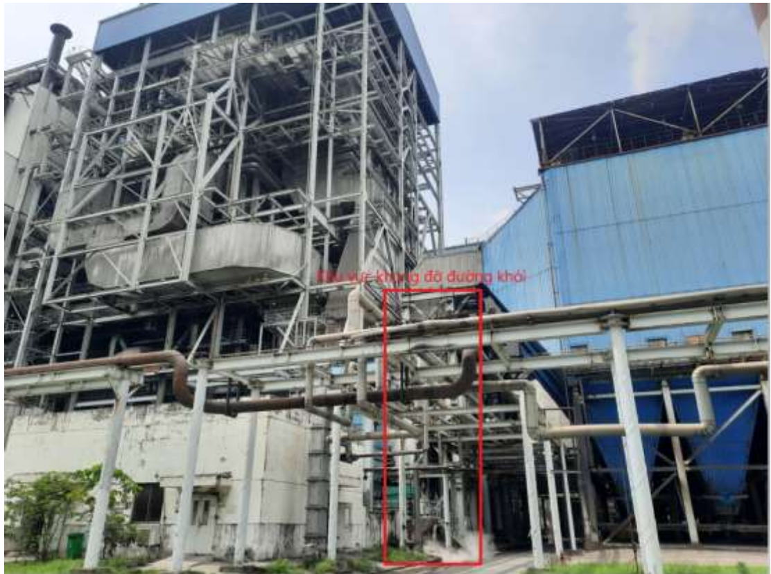
Figure 3.3: Current status image of the chimney support frame area
